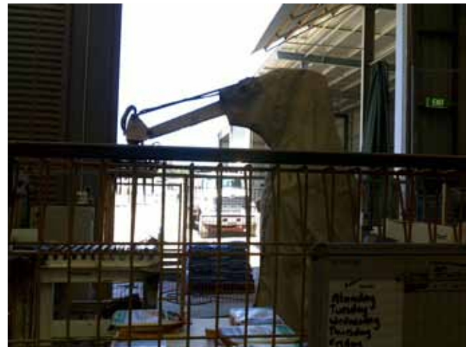
FUJI-ACE EC-101 ROBOT PALLETISER WITH DUST JACKET, SAFETY FENCING IN FOREGROUND
