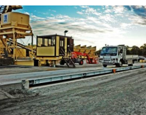
Trico Asphalt Swanbank QLD
